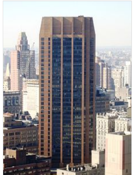
The IEEE corporate office is on the 17th floor of 3 Park Avenue in New York City.
